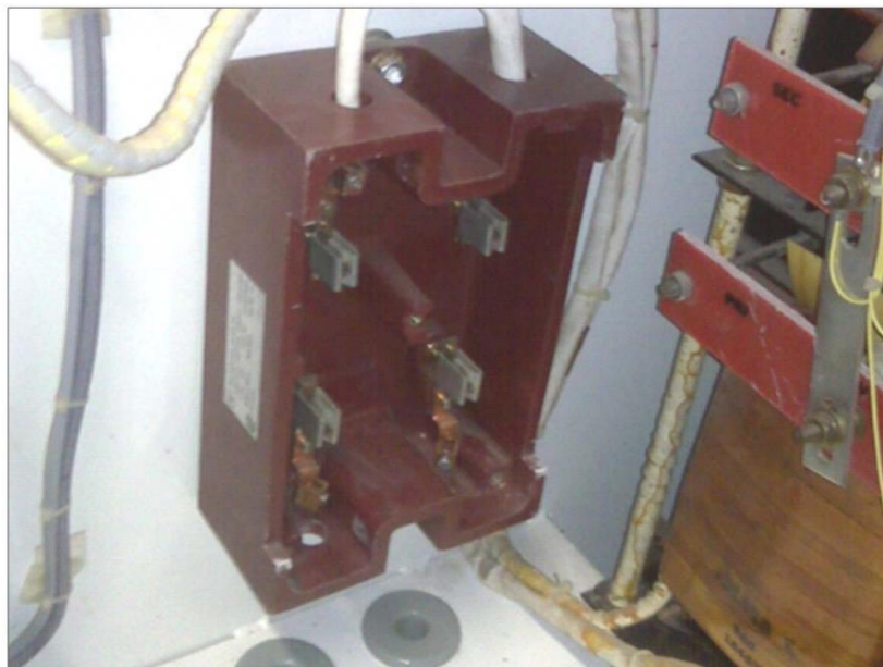
Figure 1-3. Series cut-out device receptacle (source: Liberty Airport Systems)
