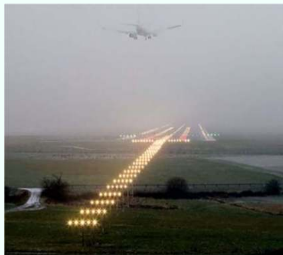
CAT I Approach Lighting System (Barrett Lights)
