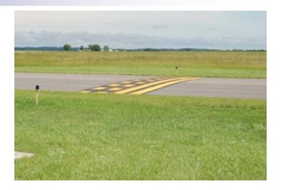
The taxiway centerline is marked with a continuous yellow line. In addition, Enhanced taxiway centre line markings, which is a Runway Incursion prevention measure, is also provided and consists of dashed lines on either side of the solid taxiway centerline.
