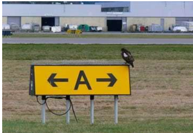
Figure 7 Deterrent Spikes don't keep all birds off of signs.
