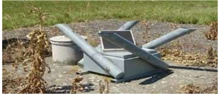
Figure 6- An underground stationary gas powered noise generator
